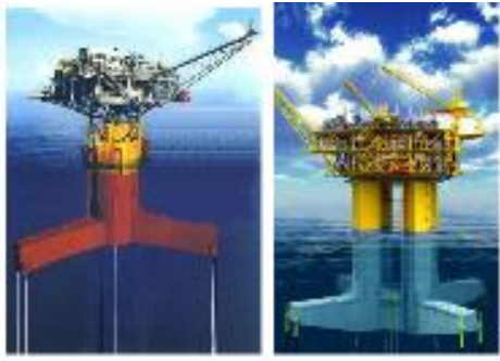
Gambar 1 Contoh Tension Leg Platform https://www.rigzone.com/training/insight.asp?insight_id=305 , 28 Maret 2022
