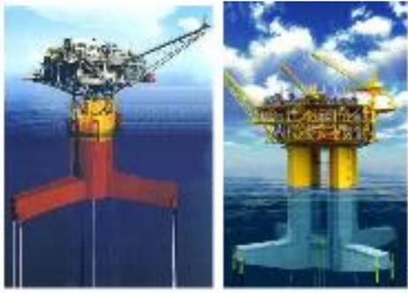
**Gambar 1** Contoh Tension Leg Platform
