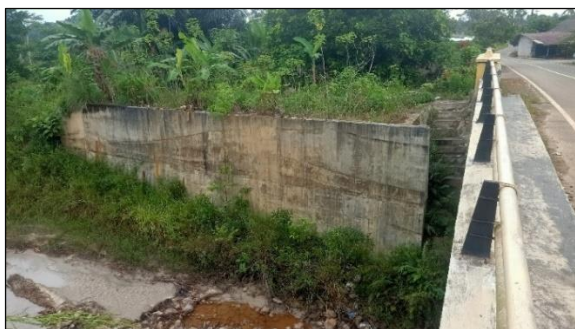
Gambar 2. Dinding Penahan Tanah Eksisting
